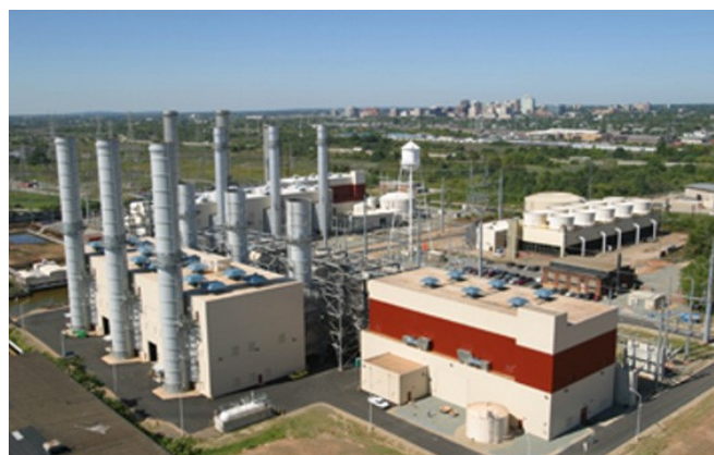
Hay Road combined-cycle plant, Wilmington, Del. (Source: Calpine)
